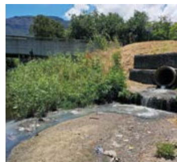
Stormwater discharged into a river, Hout Bay
